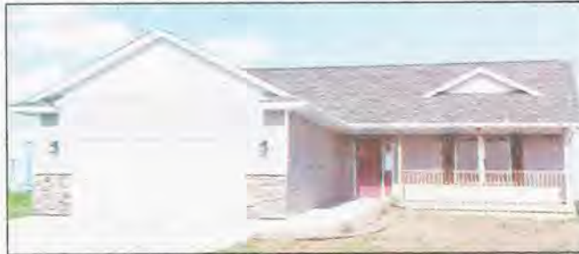
The home at 237 Peeso Creek Lane on Mondovi's north side was completed in late June and will be sold to an income-eligible family.
